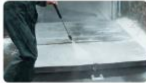
STEP 3 Rinse with water High pressure cleaner (90-150 bar, 12-30l/min.) and let dry.
